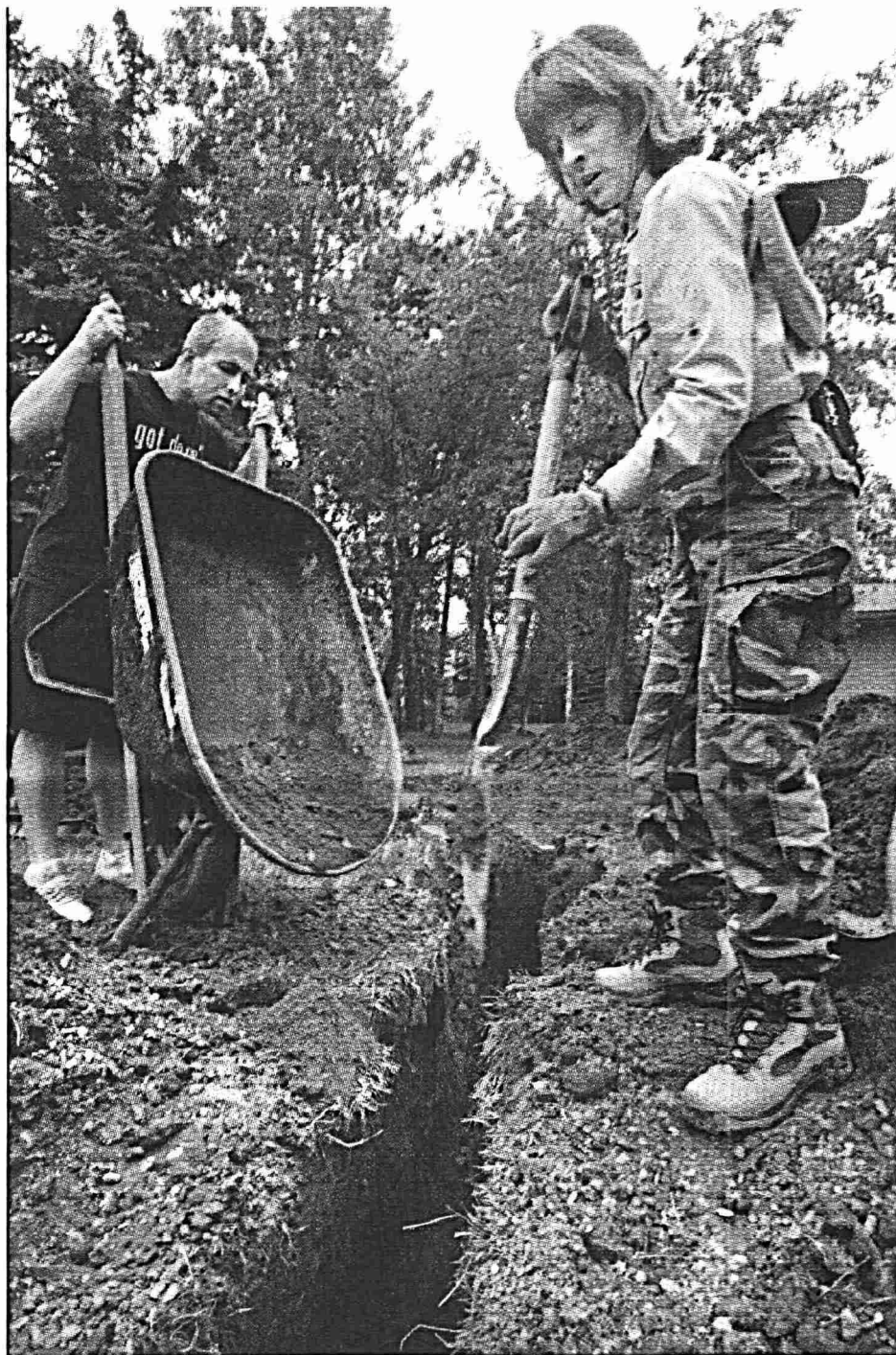
Jon Hedberg (left), a Minnesota Sea Grant intern, and Val Brady, a research assistant with the Natural Resources Research Institute , spread sand in the bottom of a rain garden's trench Thursday in Duluth's Lakeside neighborhood. The project's goal is to slow and reduce runoff and improve water quality. Photos by Steve Kuchera / skuchera@duluthnews.com
