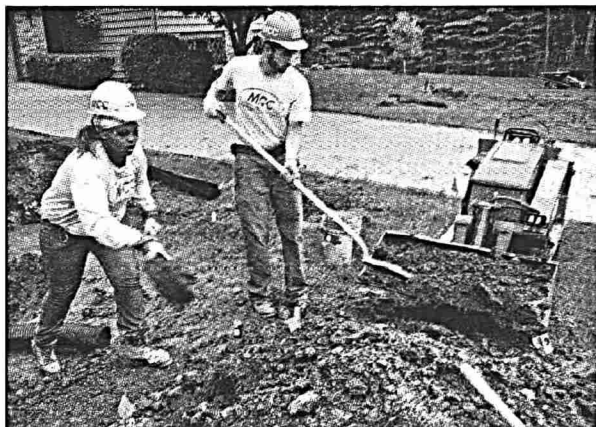
Minnesota Conservation Corps member Latasha Watson (left), 17, of St. Paul, and MCC program manager Eric Antonson remove clay from one of two rain gardens being created in a Lakeside property owner's front lawn.
